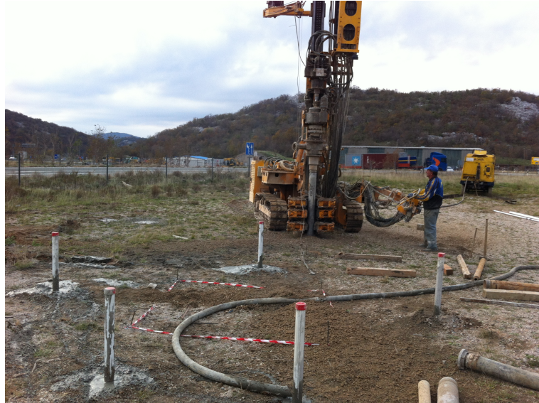
FIGURE 5.8: Drilling the inclinometer holes
