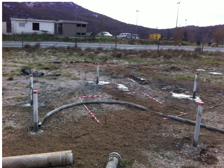
FIGURE 5.7: Inclinometer casings arranged in test field
