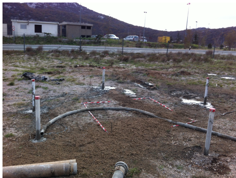
FIGURE 5.7: Inclinometer casings arranged in test field
