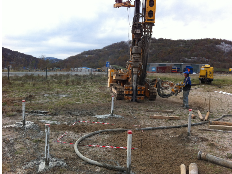
FIGURE 5.8: Drilling the inclinometer holes
