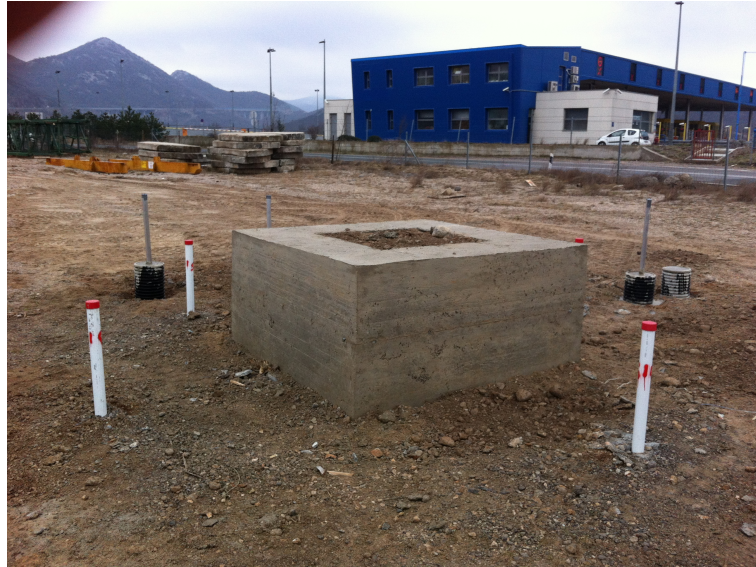
FIGURE 5.11: Completed counterweight block
