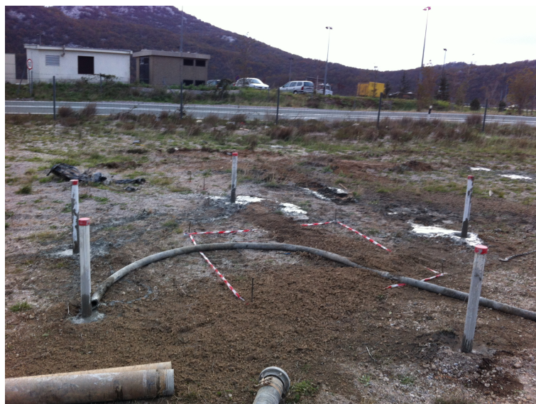
FIGURE 5.7: Inclinometer casings arranged in test field
