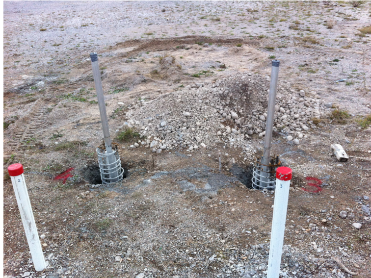
FIGURE 5.5: Pile installation
