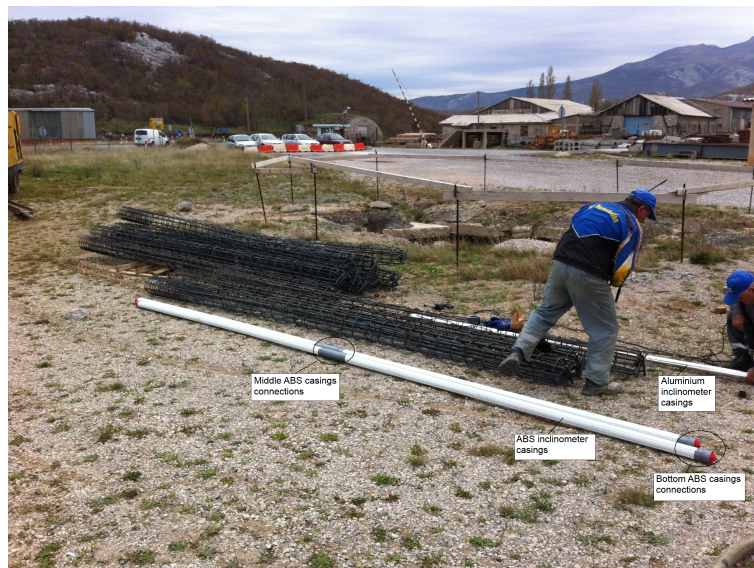
FIGURE 5.6: Six meter inclinometer ABS casings connected with ABS connection in the middle
