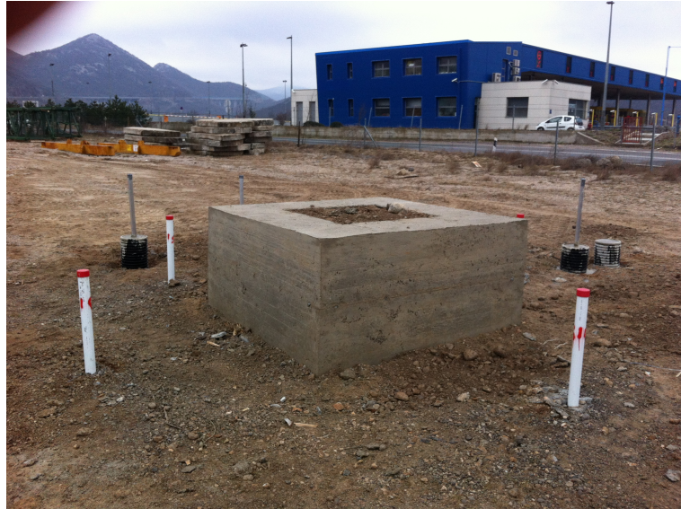
FIGURE 5.11: Completed counterweight block
